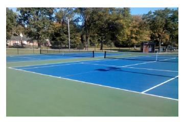
The renovations included removal of the existing artificial Omini Turf (work was done by the recreation staff). The contracted work included; 2,600 sq ft of new asphalt, expansion joint control, leveling, two coats of leveling binder filler, two coats of color, line striping, four new tennis nets, garbage receptacles and ball racks with towel holders.
